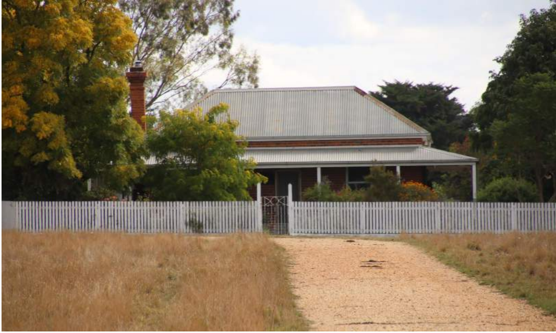
The Watts' brick homestead, Willung Road, Rosedale. 2021
